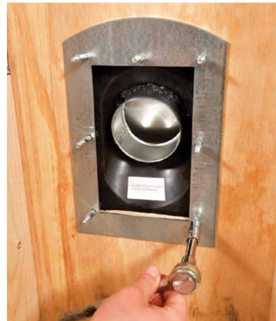
▲ The Kozy Kollar exhaust vent is easy to install, requiring seven bolts for the exhaust hood and six for the stack-pipe units. Shown here is the installation of an exhaust hood.
